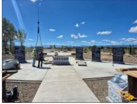
Montrose's Tri-State Generation and Transmission Assoc. crew was a big help installing the black panels, service seal stone and benches this week. PG Memorials did a fantastic job on creation and installation. Photo by Les Williams
