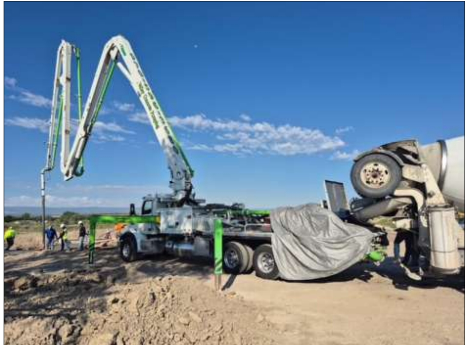
Valley Concrete Pumping in action on final pours Aug. 27, 2026. Photo by J. Bob Brueske.
