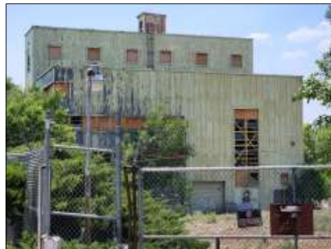
Mirror staff photo of the Bullock Electric Steam Plant taken July 5, 2026. Adjacent homeowners say that the plant has been far less secure since its purchase by the City, as the former owner had a full time caretaker and guard dog on site, neither of which exists today.
