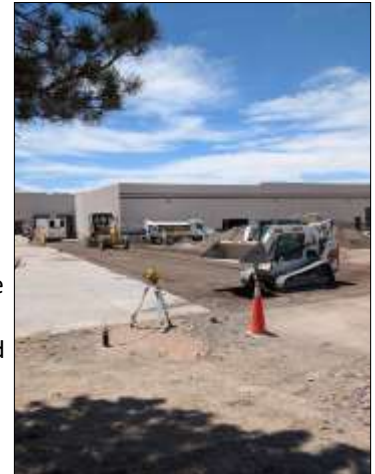
Able Excavation courtesy photo.
