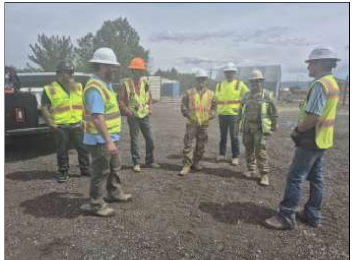
Stryker crew at work site. Courtesy photo.
