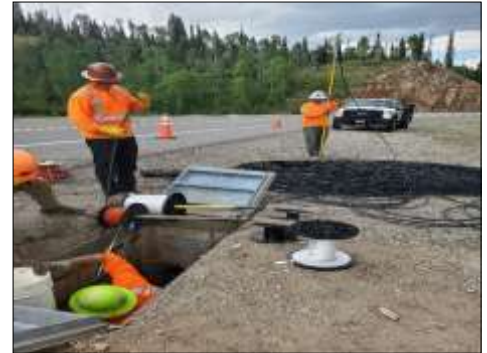
During the 2023 work season, an installation crew pulls fiber optic cable through recently buried conduit along US 160 Wolf Creek Pass east of Pagosa Springs. Courtesy photo.
