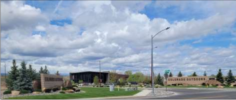
Photo of Colorado Outdoors' Mayfly Building is by Gail Marvel.
